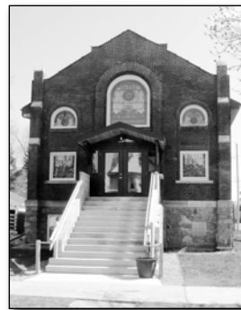
Ensure the preservation of this wonderful building.
