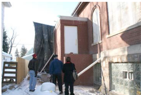
Work on the handicap lift tower
