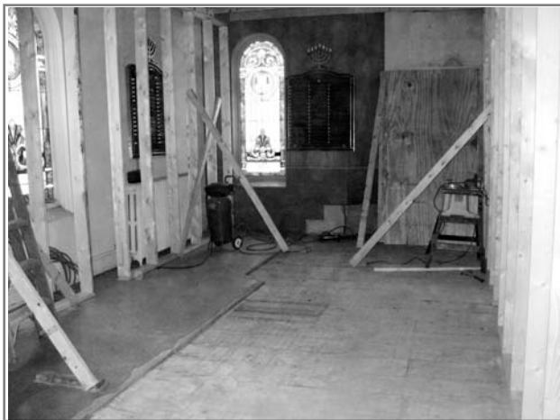
Repairs are underway at B'nai Abraham.
