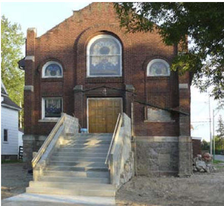
The front of the building and stairs are being historically restored.
